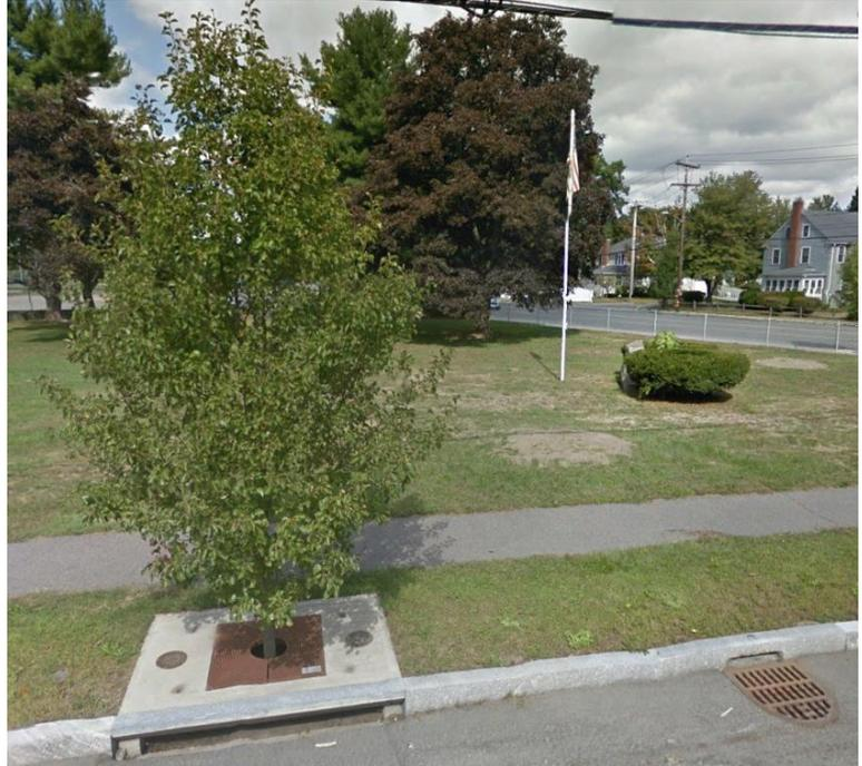
Stormwater that first runs off roadways is generally more polluted, as the “first flush” of rain washes pollutants from the street. Tree Filter Boxes capture this initial flow. When a rainstorm is large enough, the tree box will fill up; additional stormwater will bypass the Tree Filter Box and go directly to the catch basin.
