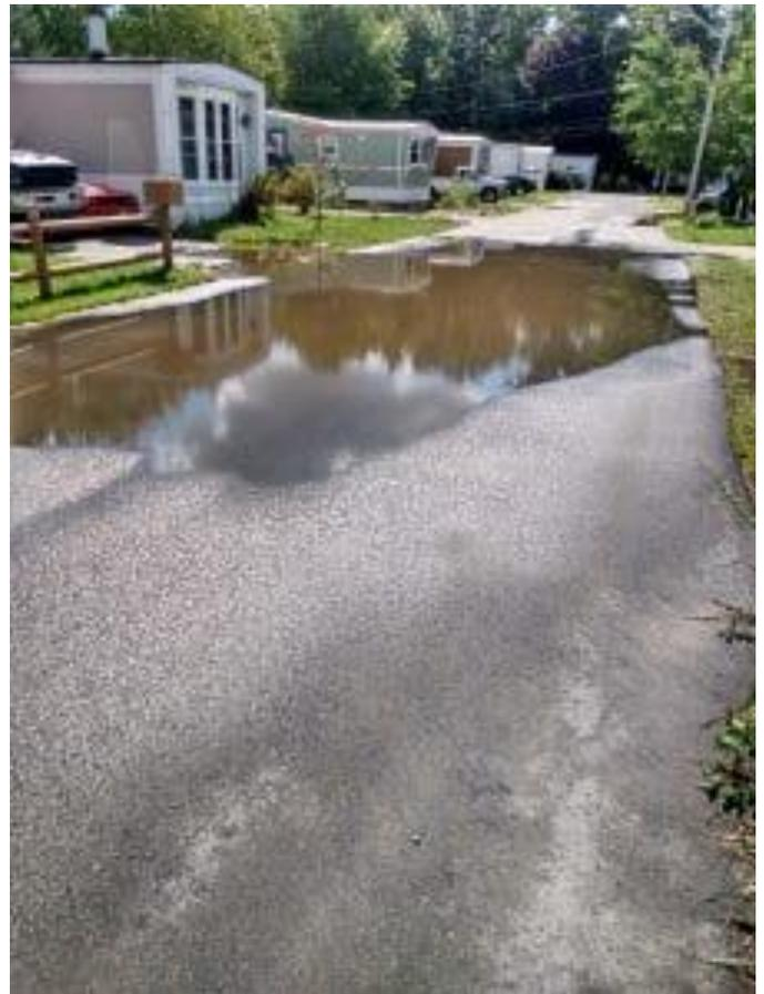
*Figure 1. Roadway flooding at the Easton Mobile Home Park after a drainage pipe was flooded by stormwater (Easton Mobile Home Owners Association).*
