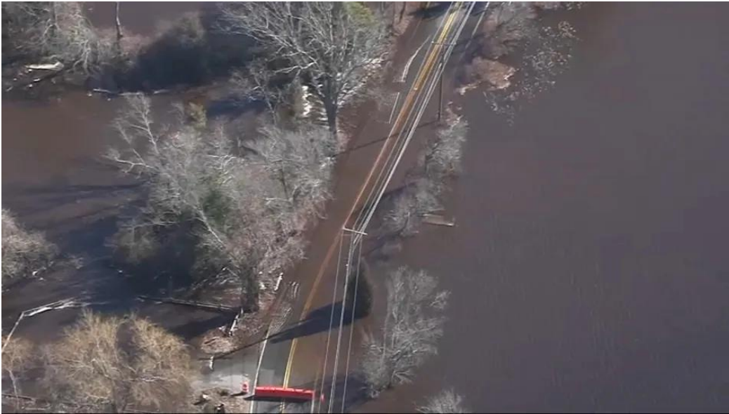
2023 Dam Breach flooded road downstream in Bridgewater Image Credit: WBZ Boston
